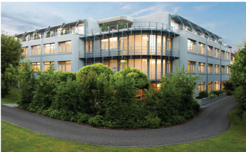
Above: Privatklinik Obach, an acute care hospital in Solothurn, Switzerland owned by Infracore SA. MPT owns a 46% interest in Infracore.
