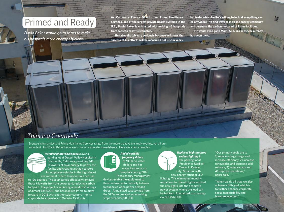
Under Baker's watch, Prime Healthcare has been installing combustion-free, solid-oxide fuel cells to take significant portions of Prime's energy usage off the power grid. It's a technology originally developed for a 2001 NASA mission to Mars. The idea was to use solar power to split water found on Mars into oxygen for astronauts to breathe, and hydrogen to power their Mars rover.
