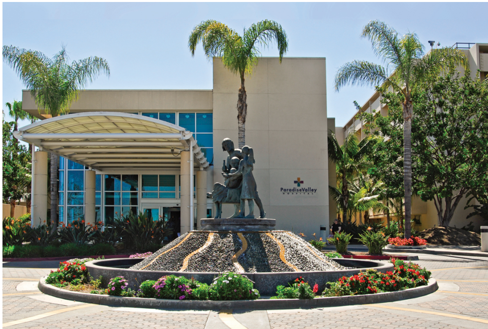
Paradise Valley Hospital, San Diego, California
